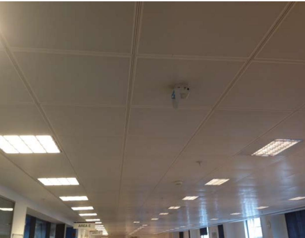
The new LED lighting is shown (on the left hand side) alongside the old T5 fluorescent fittings in the photo above taken during the course of the retrofit.
